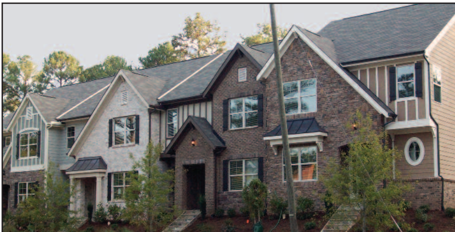
Located on Lowden Street in Raleigh's Villas at Fallon Park are 3- and 4-bedroom townhomes.
